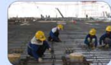
Step 8 Place reinforcement
