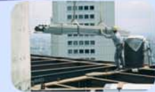
Step 1 Open SMARTDEK™ sheet bundles
